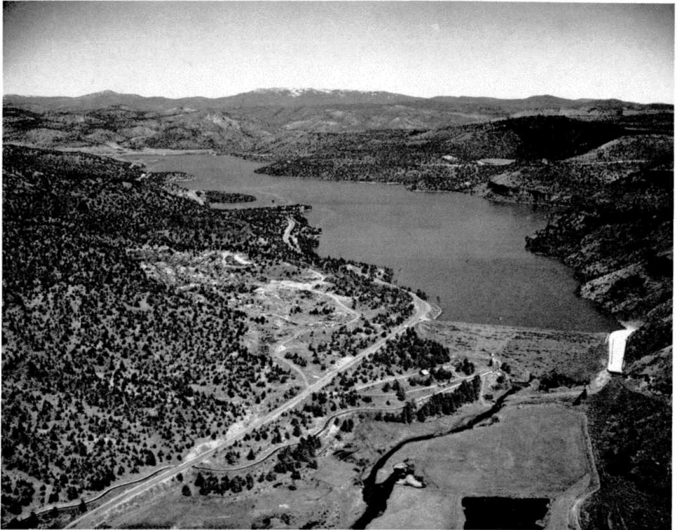
Ochocho Dam and Reservoir
